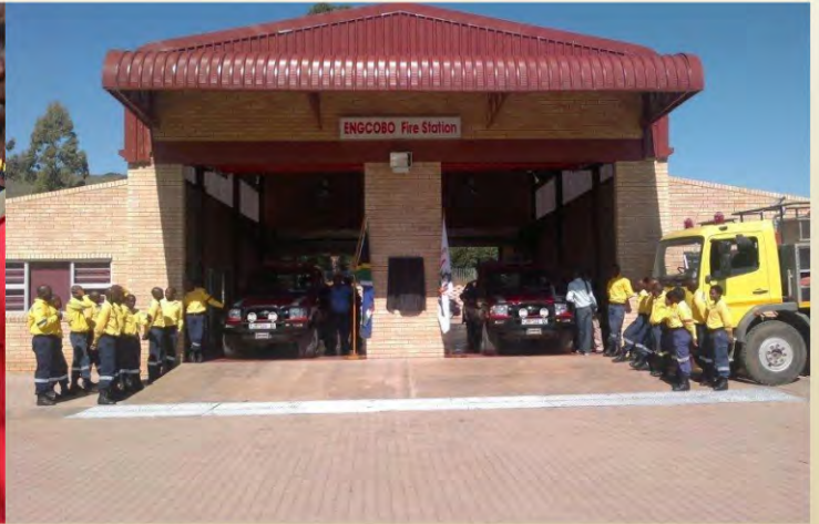
Opening of Engcobo Fire Station
