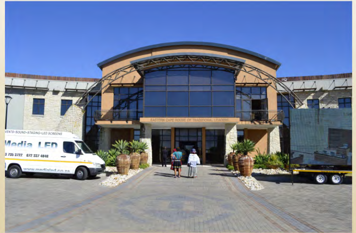
House of Traditional Leaders Building at Bhisho
