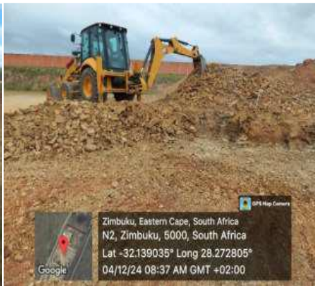
Fig 3: Excavation of cricket pitch
