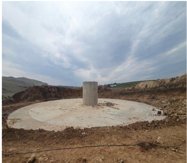
Bio-Filter Concrete Works
