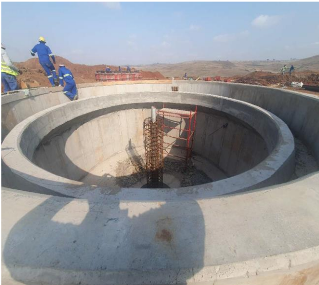
Clarifier Concrete Works
